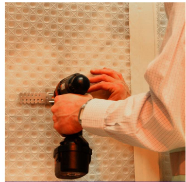
6) Screw fixing bracket to brick plug
