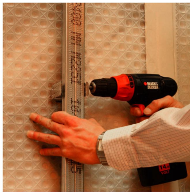
8) Secure upright to fixing bracket
