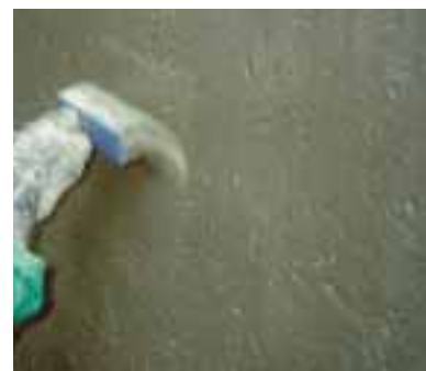
VANDEX SUPER brush application to inner concrete wall surfaces
