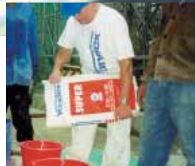
Mixing of VANDEX SUPER
