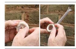
Ensure the flange of the Stormdry Gauge is clean and dry, and then apply mastic adhesive. Complete an "O" ring of adhesive, ensuring there are no air gaps.
