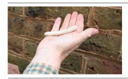
Peel back the release paper from the mastic adhesive, and roll between hands. A length of approximately 10cm (4") is required to create a complete seal around the flange on the Gauge.
